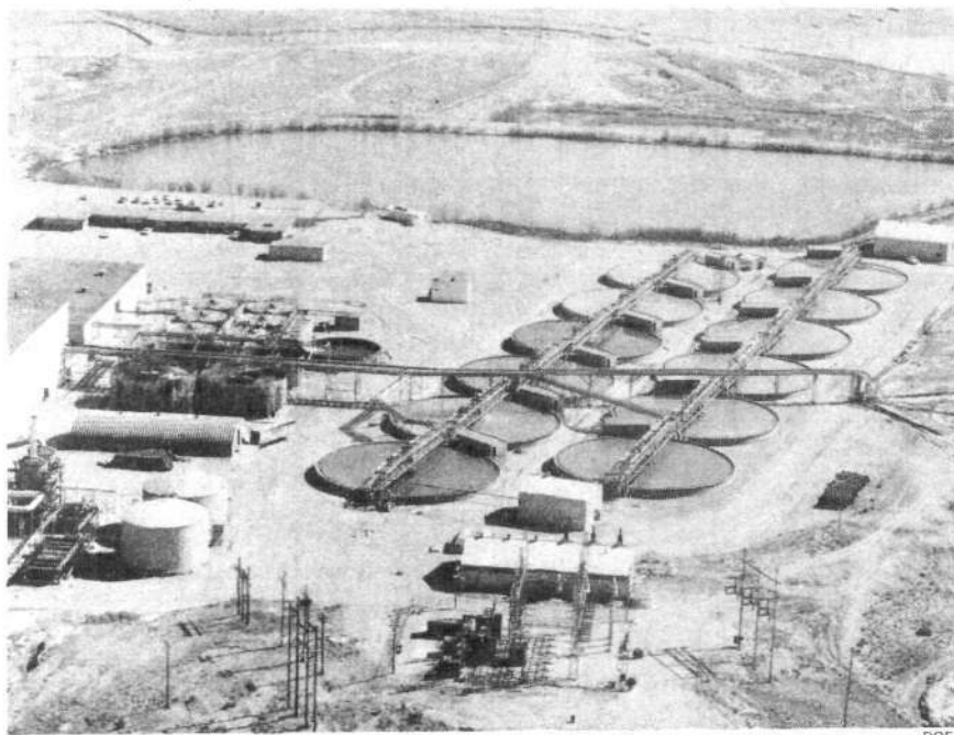
The thickener section of a uranium mill in New Mexico's Grants uranium belt, the single largest reserve in the United States.
