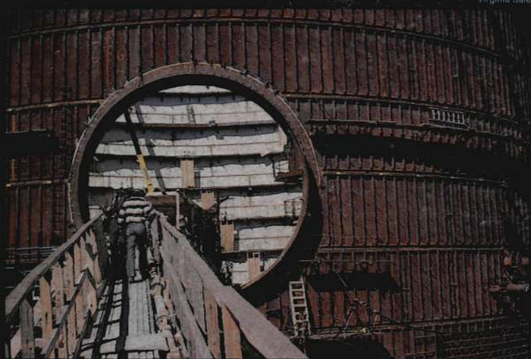
The containment vessel of the Seabrook, N.H., nuclear plant under construction.
