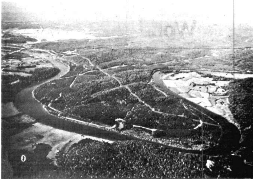
Aerial view of the site of the Clinch River fast breeder reactor in Oak Ridge, Tennessee. ERDA
