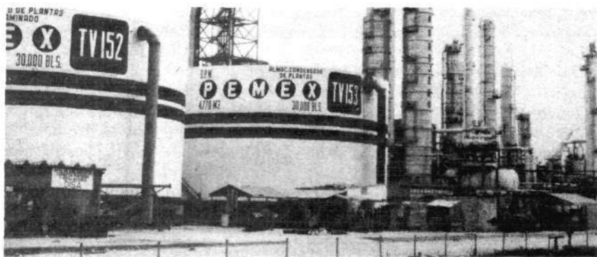
Reduced oil revenues may force cutbacks in Mexico's capital goods imports. Above, the Pemex petrochemical facility in Veracruz.
