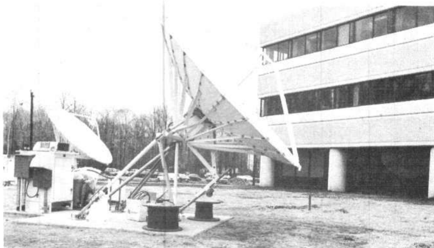
A new satellite communications system links up the National Magnetic Fusion Energy Computer Center at Lawrence Livermore with the Plasma Physics Lab at Princeton. This is the first of a number of planned linkups that will enhance the U.S. magnetic fusion program.
