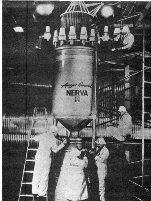
NASA This full-scale mockup of the Nuclear Engine for Rocket Vehicle Application (NERVA) allowed engineers to observe component orientation and limitations on spatial arrangement. The mockup was constructed by Aerojet-General Corp.
