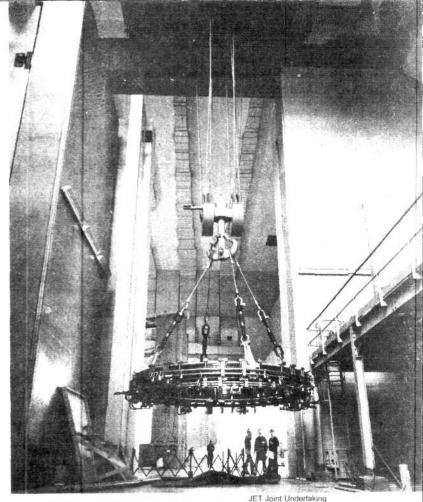
One of JET's poloidal field coils being transported into the Torus Hall at Culham Laboratory.
