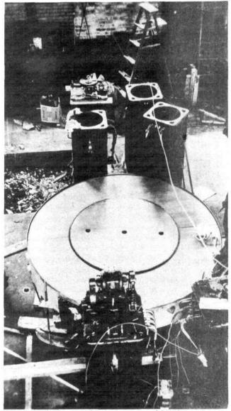
"We built the best cyclotron in the world." Shown here is the cyclotron core (50 inches diameter) as the magnet and coils were being assembled.
