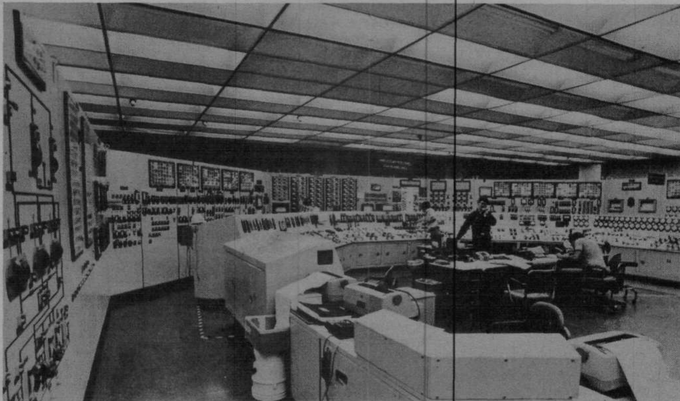
The Unit 2 control room during normal power operation in early 1979. The plant is highly automated and when things are running normally, the operators primarily monitor instruments.
